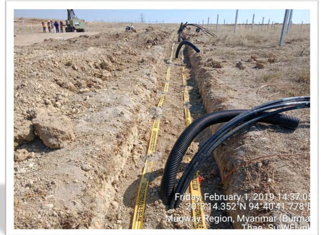
BACKFILLING OF DC CABLE LAYING
