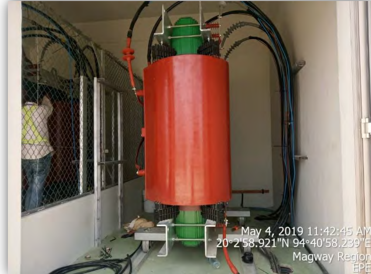
33/11kV, 2MVA Transformer
