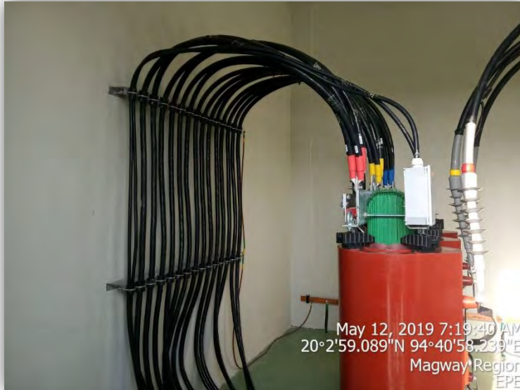
11/0.4kV, 500kVA Transformer
